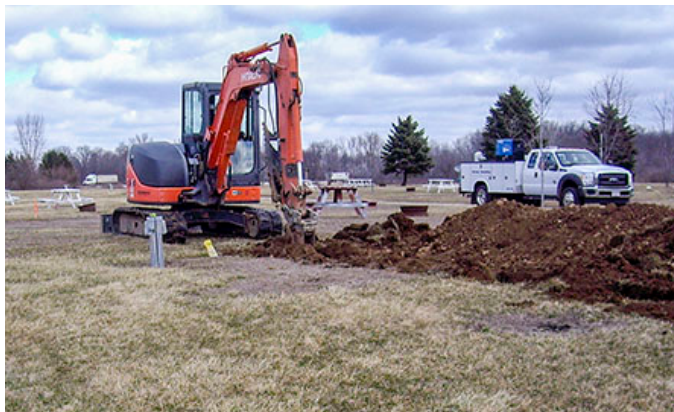
Working on our electric upgrade
