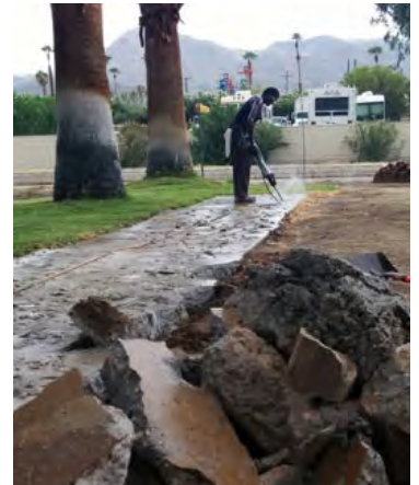
Travis breaks up a concrete to make more room for campfires
