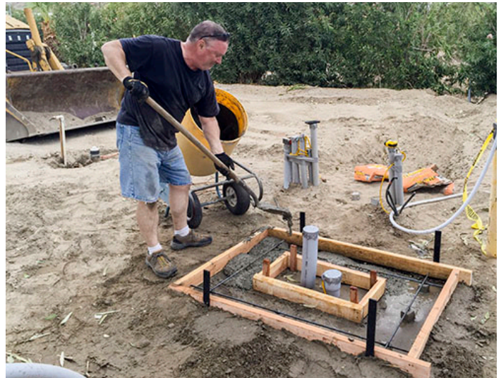
Mike preparing one of the transformer pads
