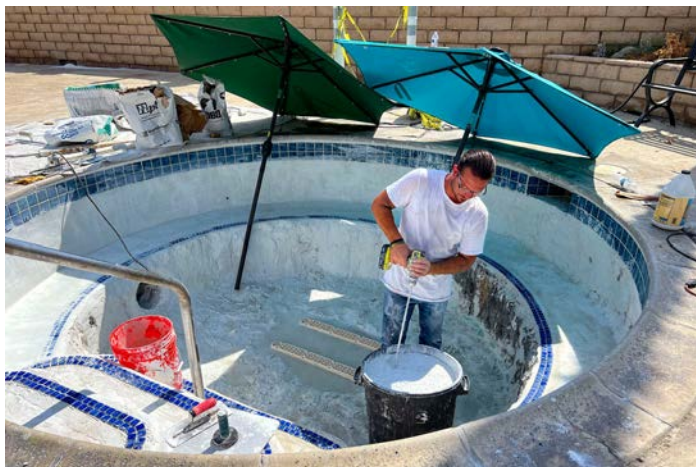
Replastering the spa almost complete
