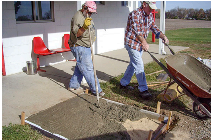
Dave and Gary working on the wheelchair ramp
