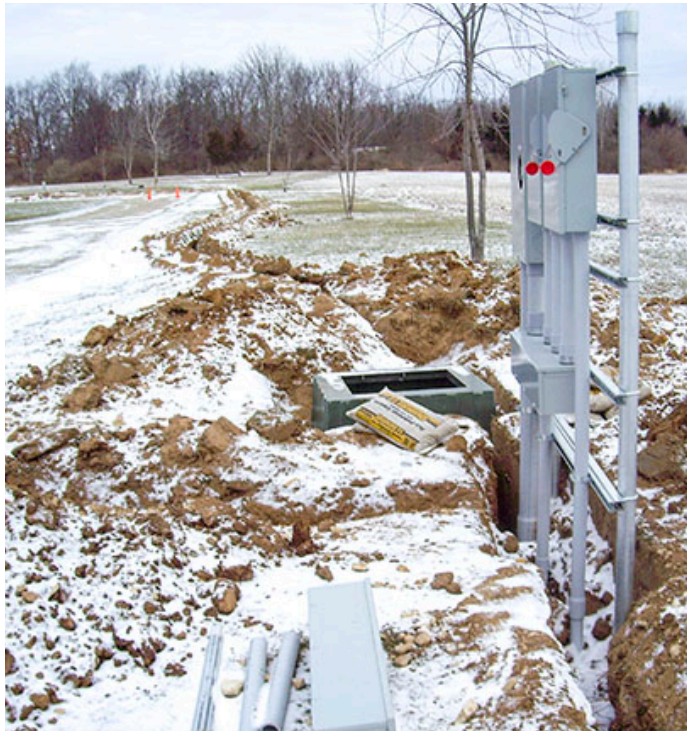
Despite the cold weather, work continues on the electrical upgrade
