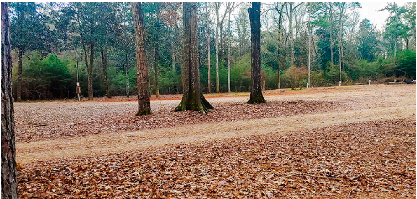
With the old kitchen demolished and removed, we've made room for new RV sites
