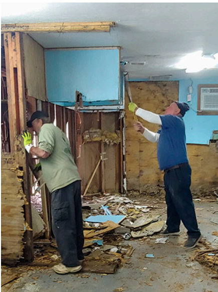
Bath house renovation
