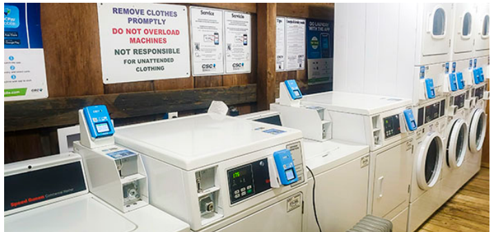
All new laundry room
