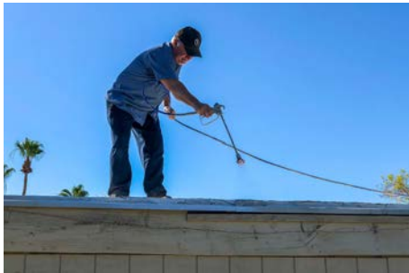
Mike sealing the kitchen roof
