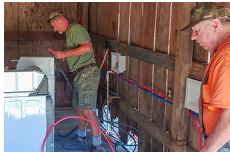
Scott and Charles working on the temporary laundry
