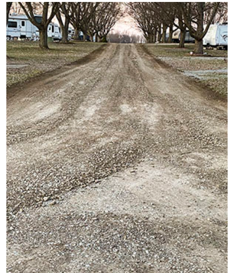
Ongoing road widening
