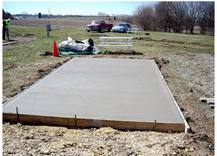
One of the new pads
