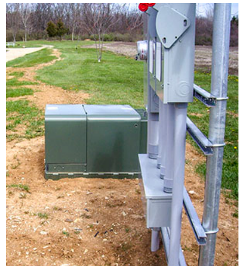
New electric upgrade
