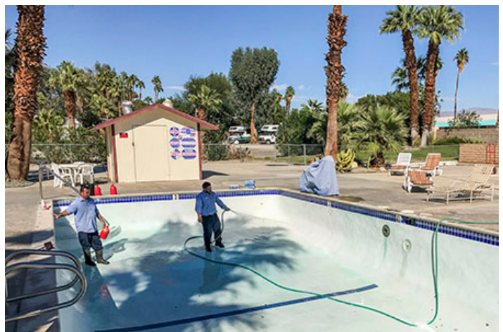
Acid wash of the pool in progress...
