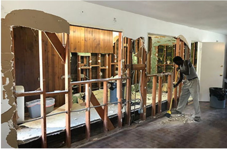
Travis cleans up after the first round of demolition
