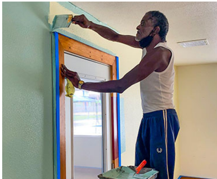
Travis painting the lobby
